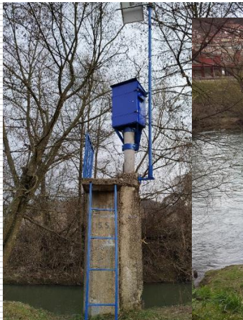
Hydro. staton Zavlaka The Jadar River
